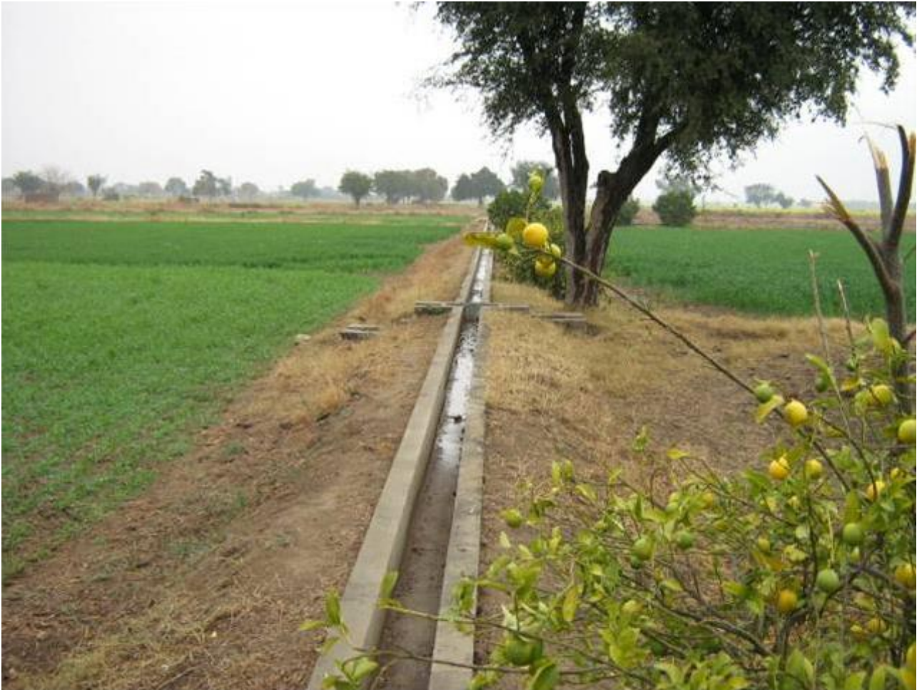
picture: irrigation drain
